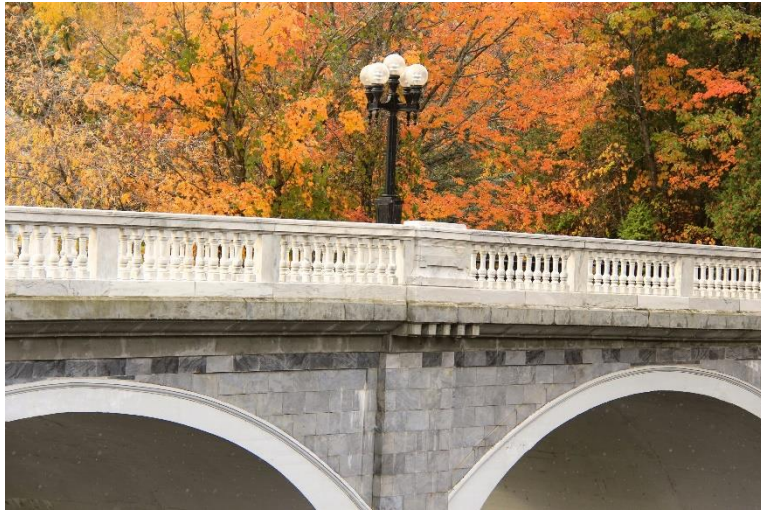
Image: Proctor's Marble Bridge. Source: Dale Christie
