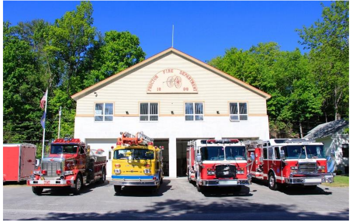
Image: Proctor Town Fire Station. Source: Dale Christie.
